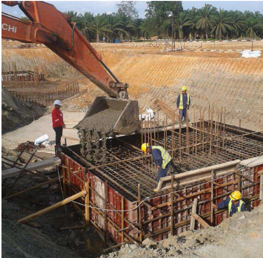
First concrete pour on furnace foundation in April 2014
