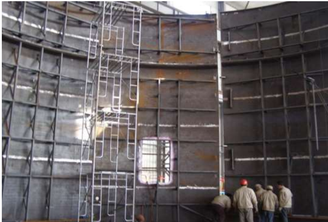
Inspection of Furnace shell during trial assembly in China
