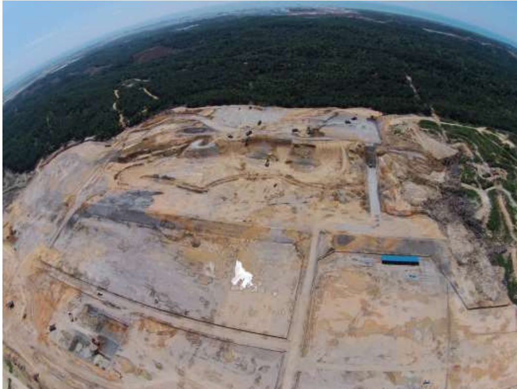
Project site aerial view as at end April 2014
