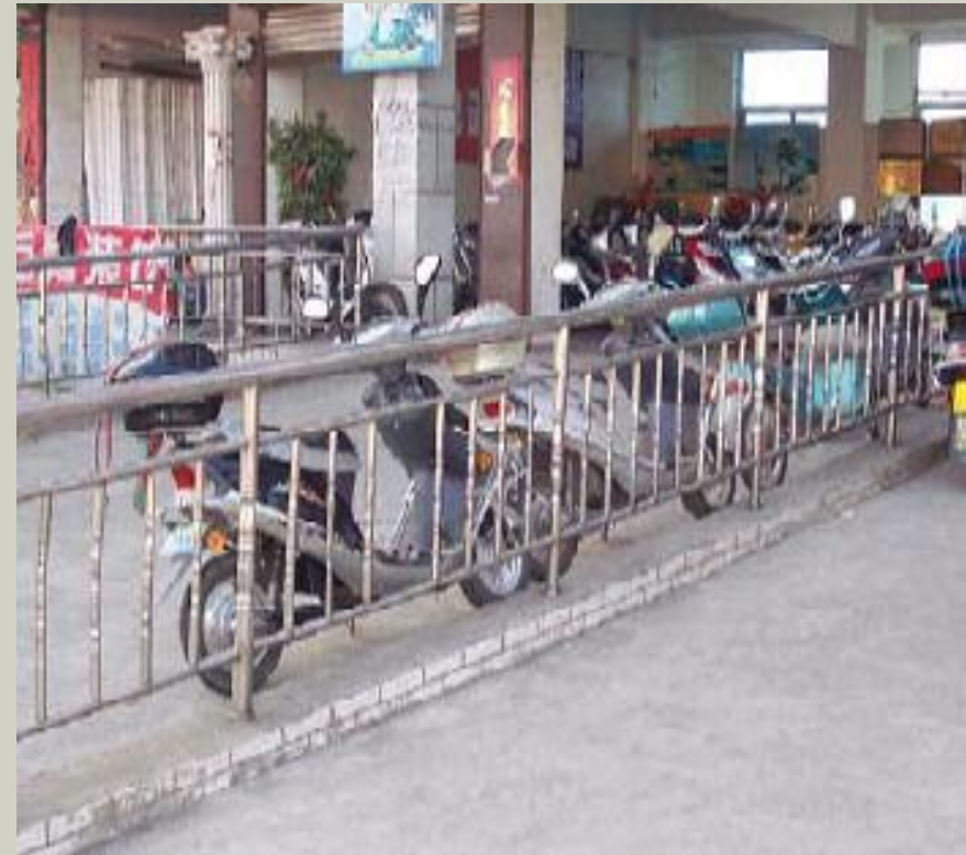
Structural tubes - handrails
