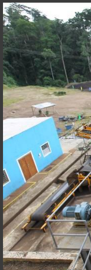
选矿现场 The Scene of Ore Dressing Plant
